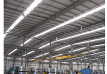
This manufacturing facility at Emu Plains uses roofing and walling specially rollformed from COLORBOND® steel in thickness 0.6mm BMT. Roofing profile is LYSAGHT KLIP-LOK 700 HI-STRENGTH®.
